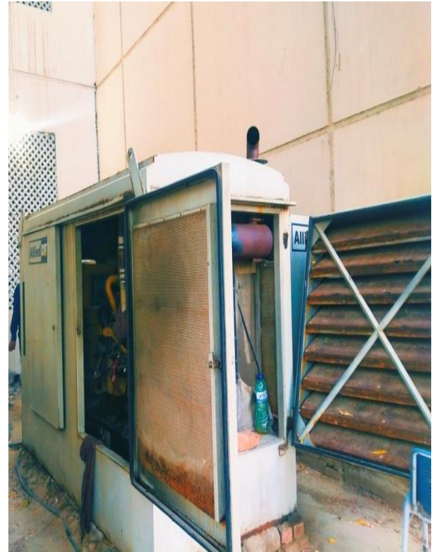
Figure 3. 50KVA diesel generator at Hostels
